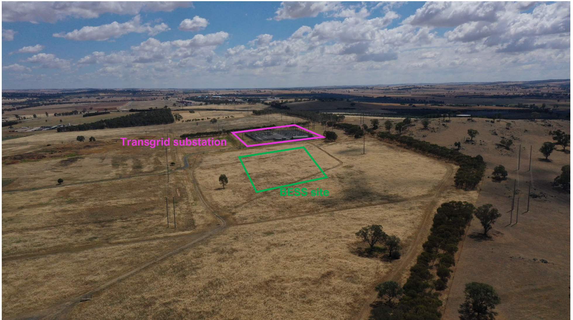
Figure 4-15 View of proposed development site as cleared cropped land (Source: Ember, 2024)
